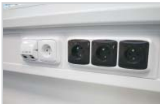
Example of installing the PK 140X70 D parapet trunking.
